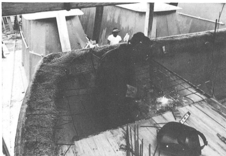
Water tank top reinforcing.
