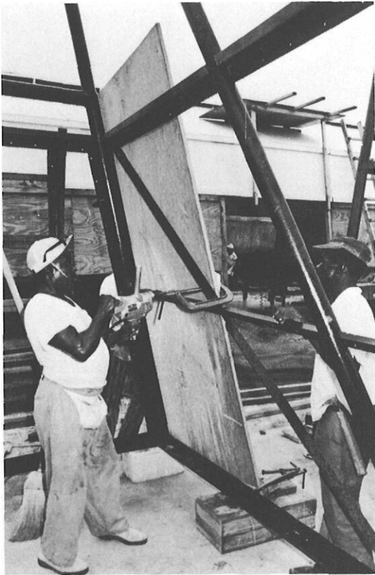
Drilling holes to secure the plywood for marking.
