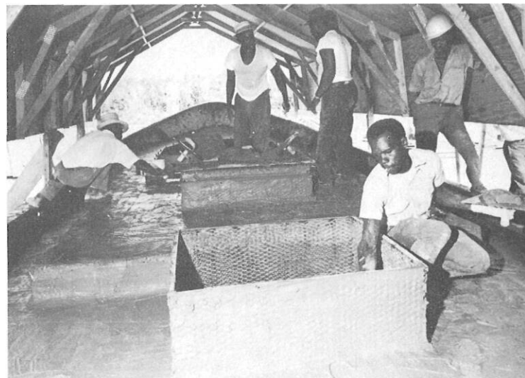
Plastering coaming from inside.
