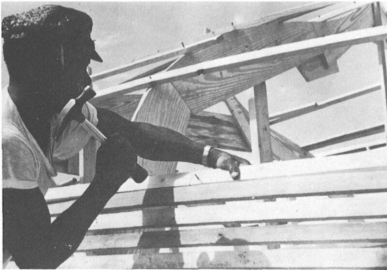
Splicing a plank.
