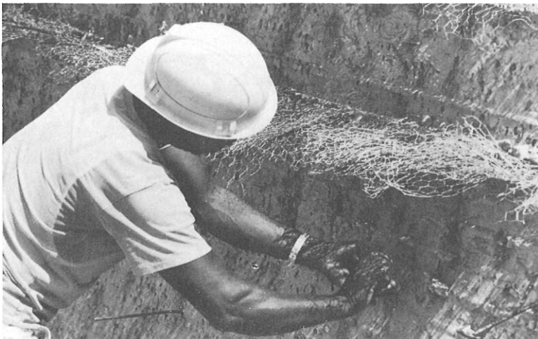
Clipping off staple ends in awkward places.
