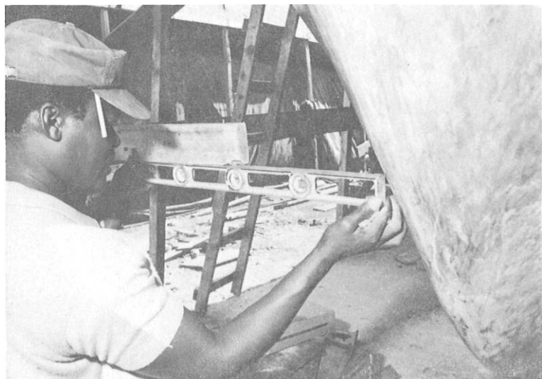
Transferring waterline marks from the shelter face to the hull.
