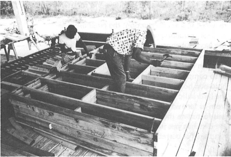
Series assembly of fish-hold frames.
