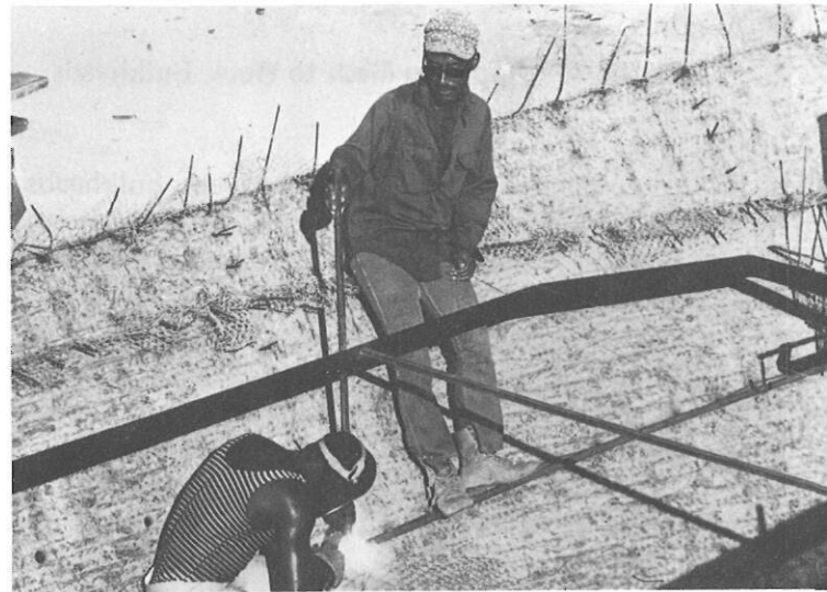
Aligning wheelhouse base frames.
