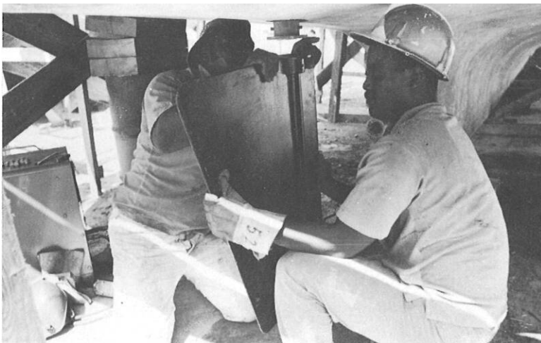
Matching flange on two-piece rudder stock.
