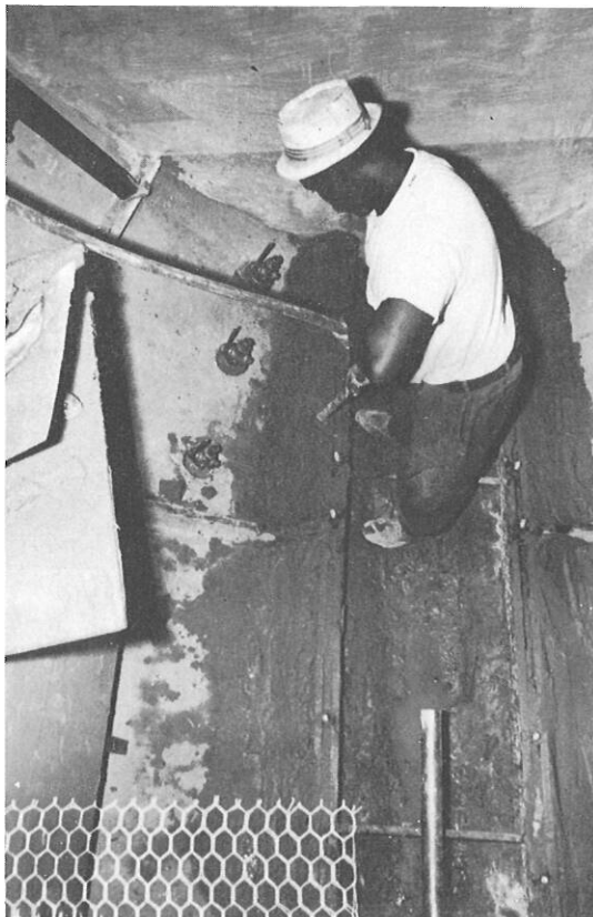
Vibrating mortar into engine beds.
