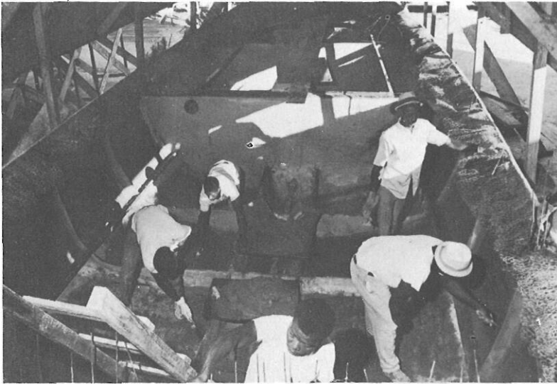
At work on interior skim coat.
