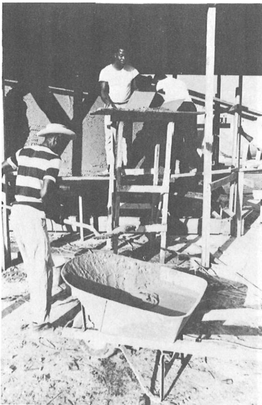
Into buckets and up onto the mortar board.
