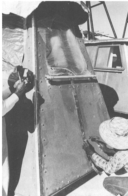
Nailing protective copper strips over joints.
