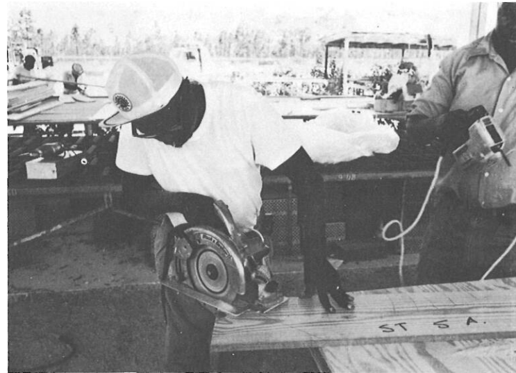
Saber and rotary hand power saws were used to cut the boards.
