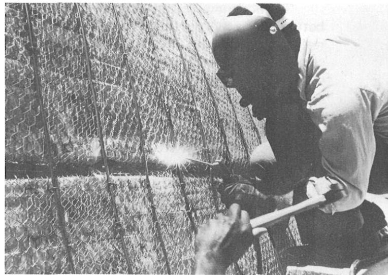
Welding the deck starter rods.
