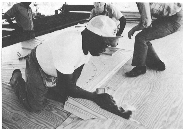
Trimming to fit center line.
