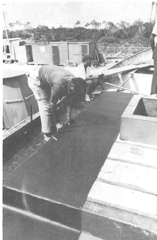
Tarpaper being stapled over deck mold.
