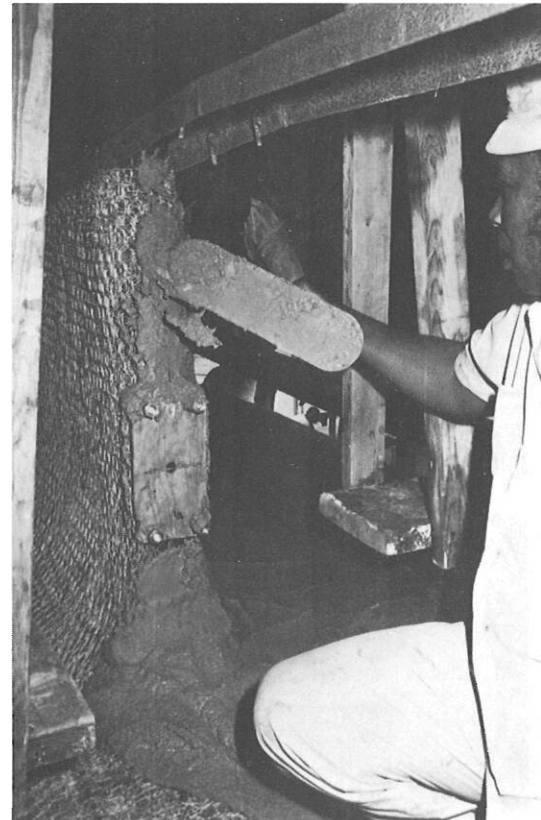
Applying mortar to the stern post. Note suspended scaffolding.
