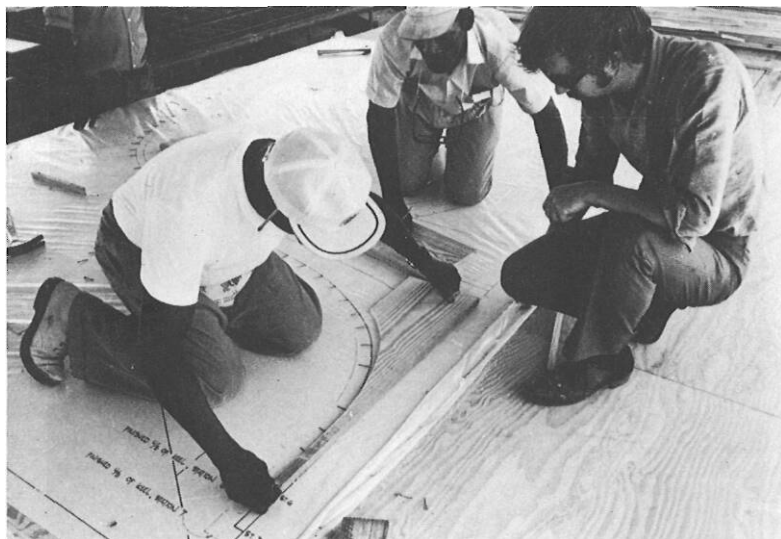
The cut boards are checked against the pattern lines.
