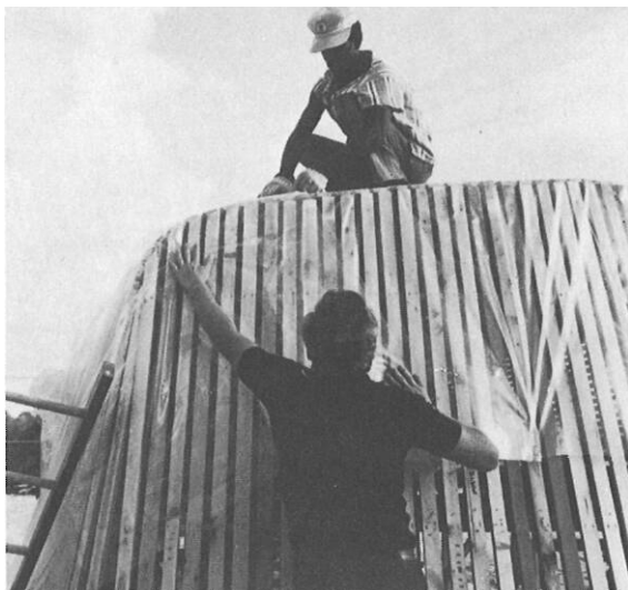
Plastic sheathing is stretched taut and stapled.
