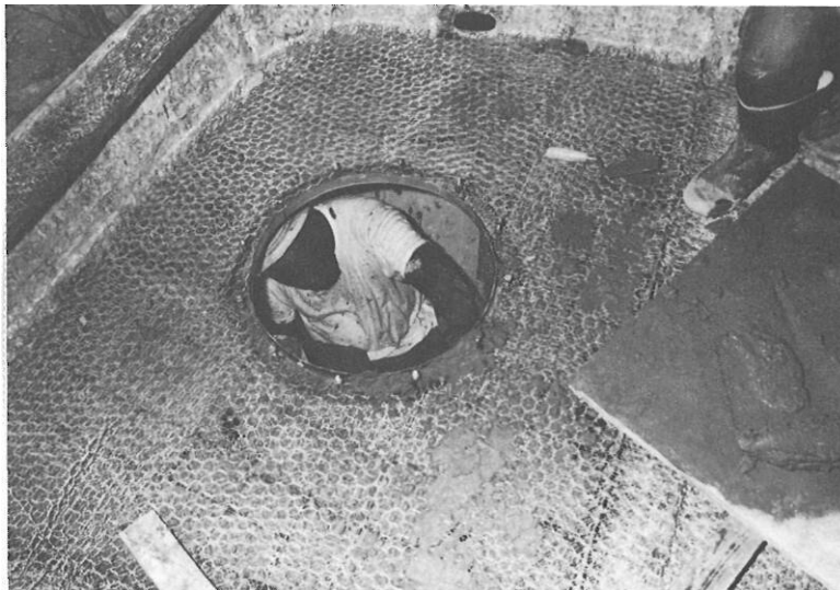
Plastering water tank interior top.
