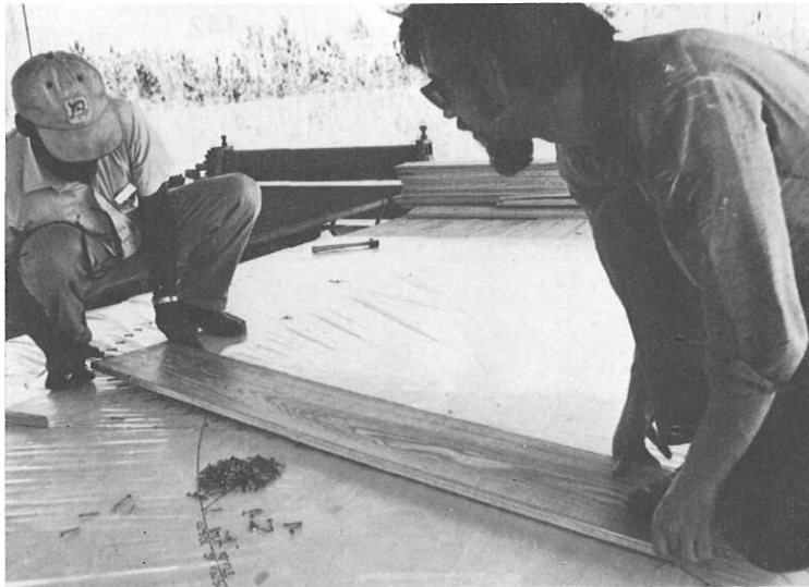
The board to be cut being laid over the nail heads.
