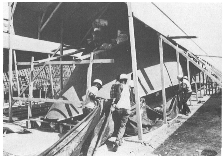
The steam tent being hauled to yesterday's plastered hull.
