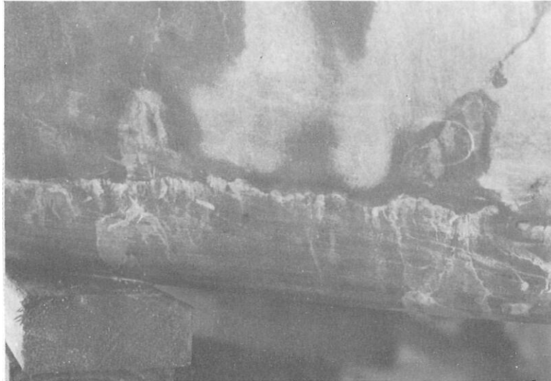
Sodium silicate forming a seal.
