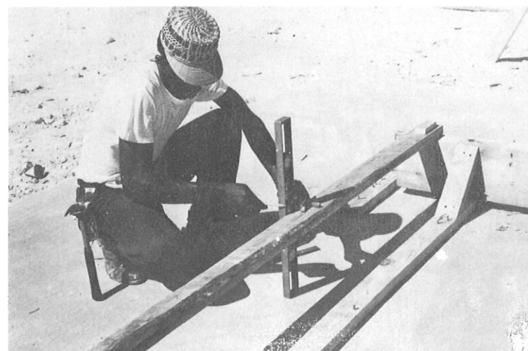
Establishing the center line.
