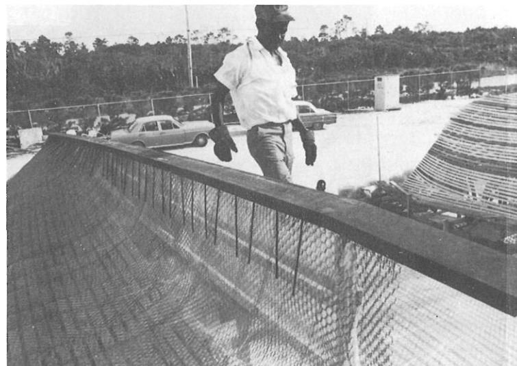
Keel shoe laid in place.
