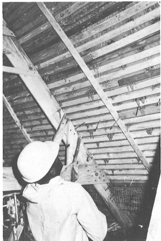
Well vibrated mortar seeps through the weld bums in the plastic sheeting.
