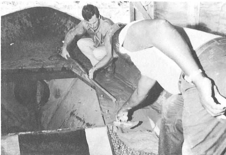
John Samson demonstrates use of vibrator on the deck.
