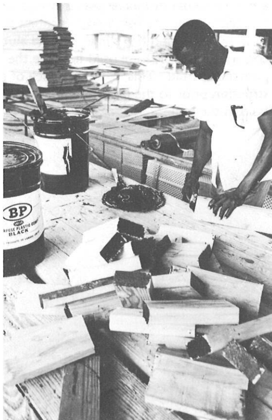
All joints treated with waterproof compound.
