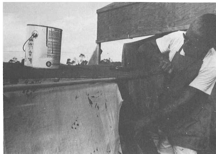
Priming the molding.
