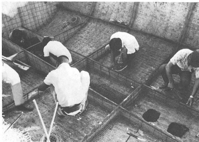
Holes punched through the skin above the deadwood cavity, to be filled with mortar later.
