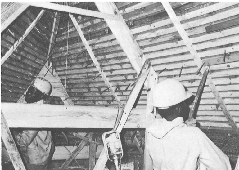
Vibrating along the planking and checking the gaps for penetration.
