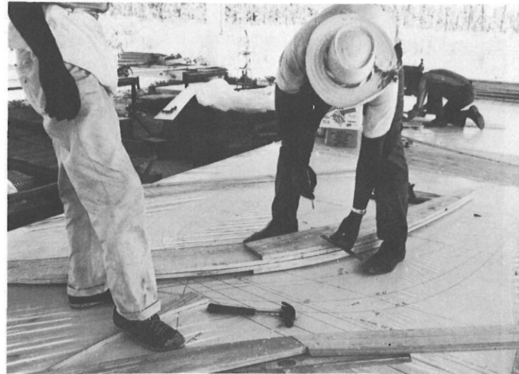
Two half frames assembled at once. Note position of scabs.
