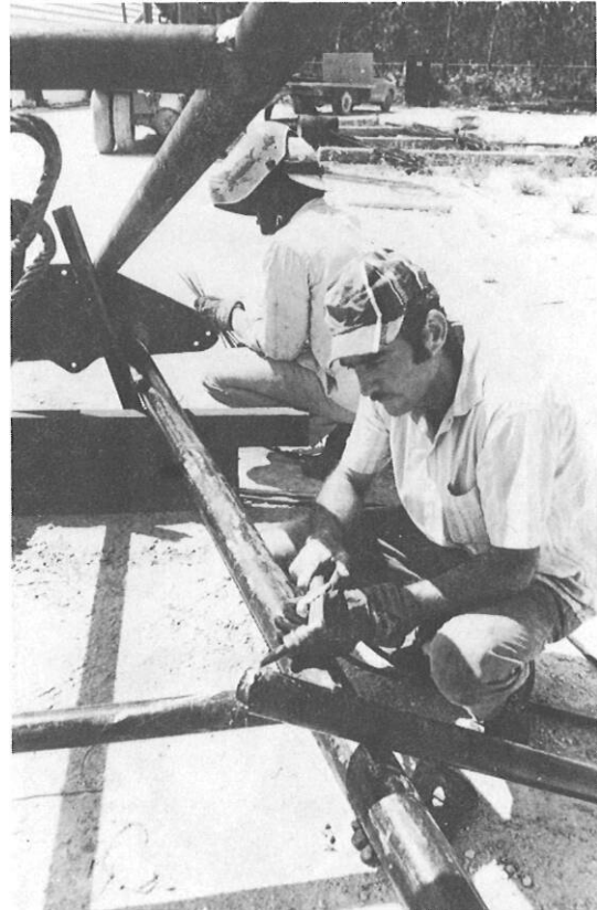
Bracing and assembling the two A-frames.
