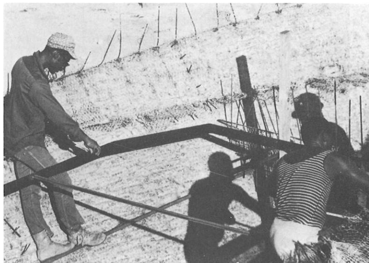
The base frame must be level and true.
