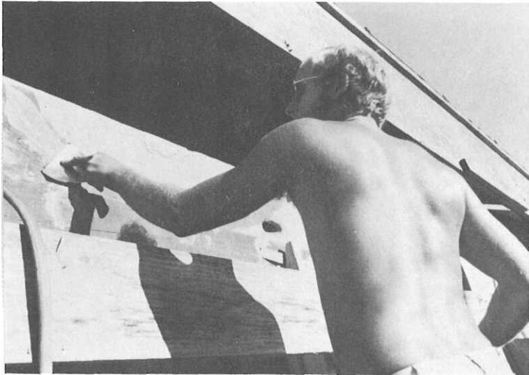
Filling the cracks.
