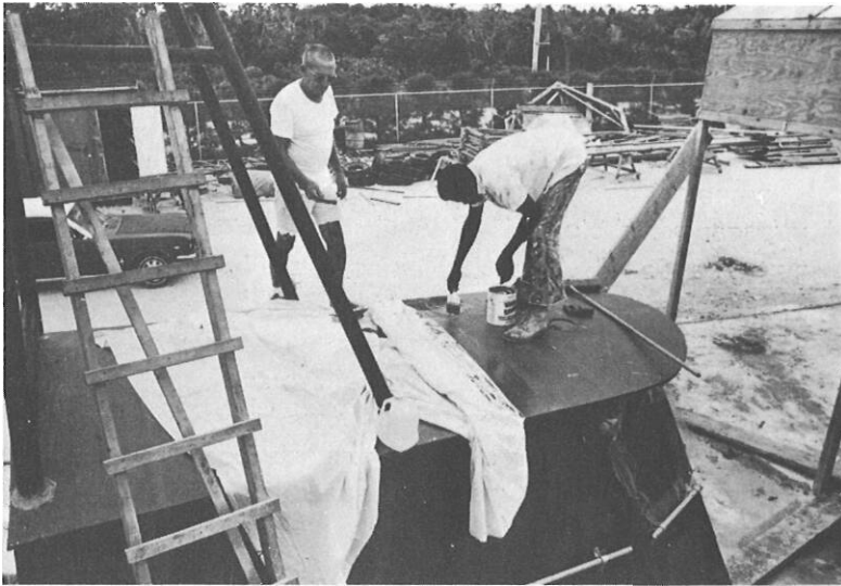
Sealing the roof with second coat of red lead paint.
