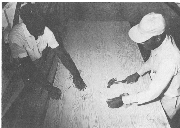
Nailing the frames down.
