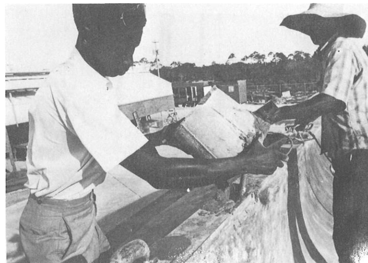
Pouring and vibrating.
