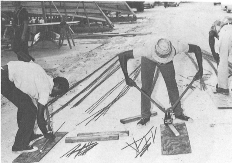
Cutting starter rods.
