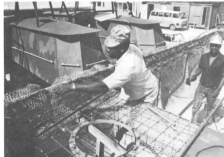
Rail cap rods leveled, screed goes on.
