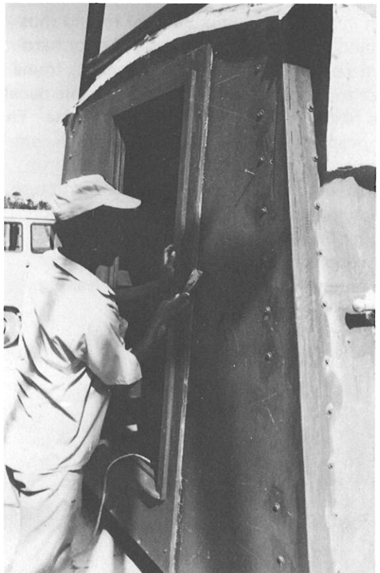
Removable aft panel tacked into position prior to bolting.
