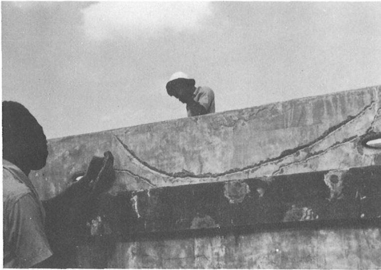
Cracks being chipped open for repair.
