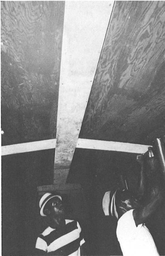
Butt blocks glued and screwed to the roof interior.
