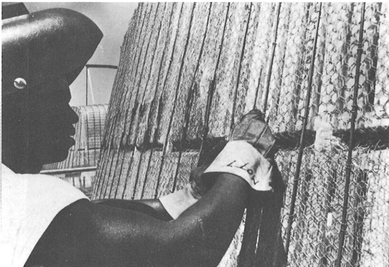
Welding deck starter rods.
