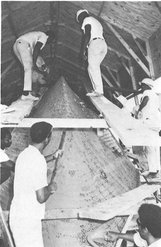
Pencil-type vibrator being used on the stem.
