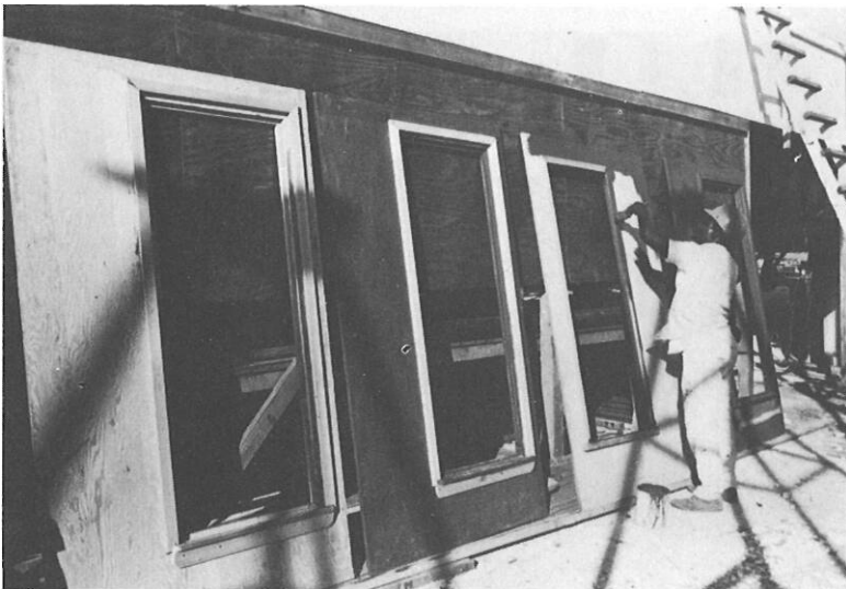
Removable aft panels with door frames fitted.
