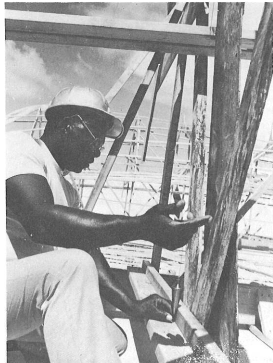
Checking plumb of keel.
