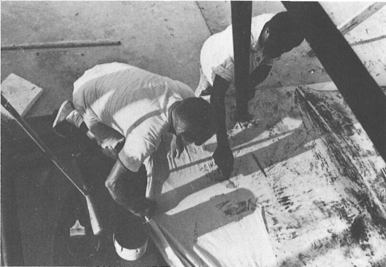
Stretching the cloth over fresh paint.
