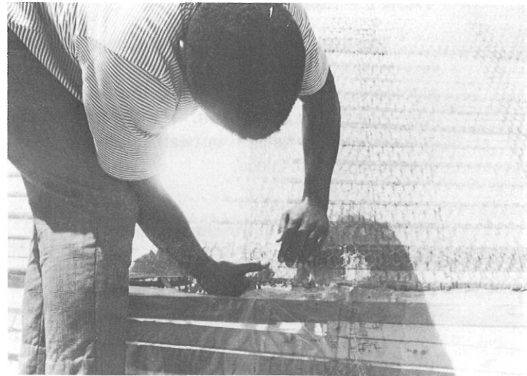
Tucking surplus mesh into the deck cutout.
