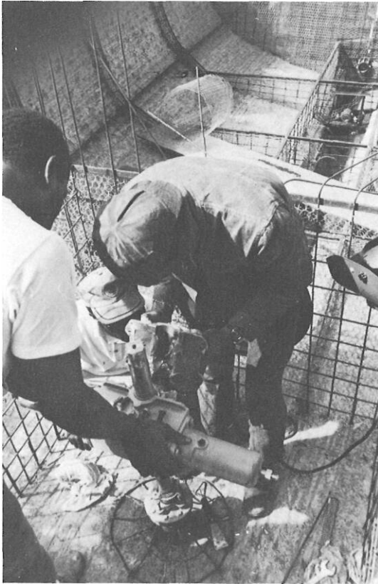
Cone-shaped reinforcing to stuffing box housing.
