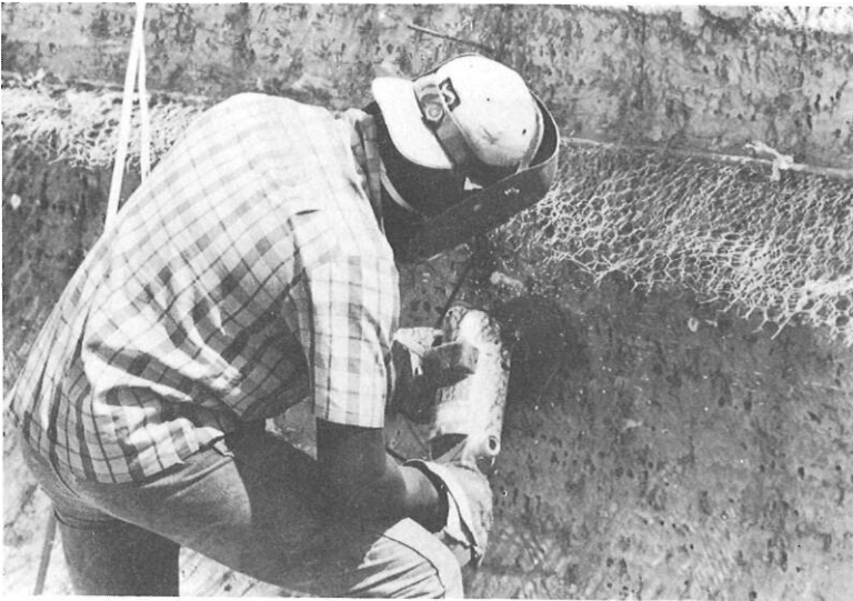
Grinding off the staple ends.
