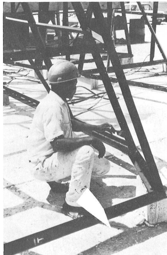
Touching up scratches with coal-tar epoxy.
