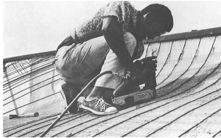
Stapling the vertical rods down with air-powered staple gun.
