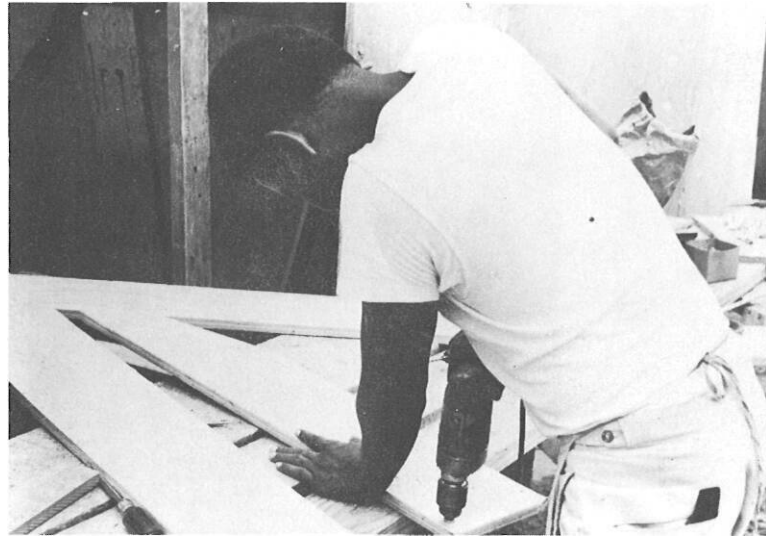
Preparing plywood butt blocks.
