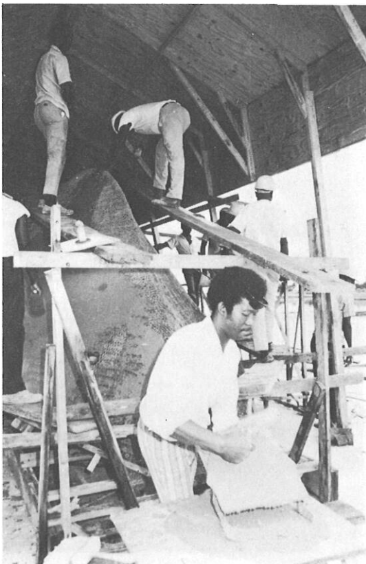
Trimming the loaded hawk.
