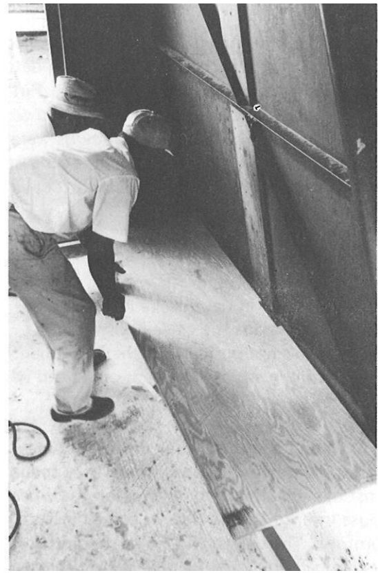
3/4-inch (19 mm) plywood flooring.
