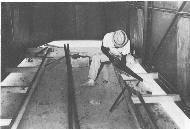
Sawing packing for outside edges of floor.
