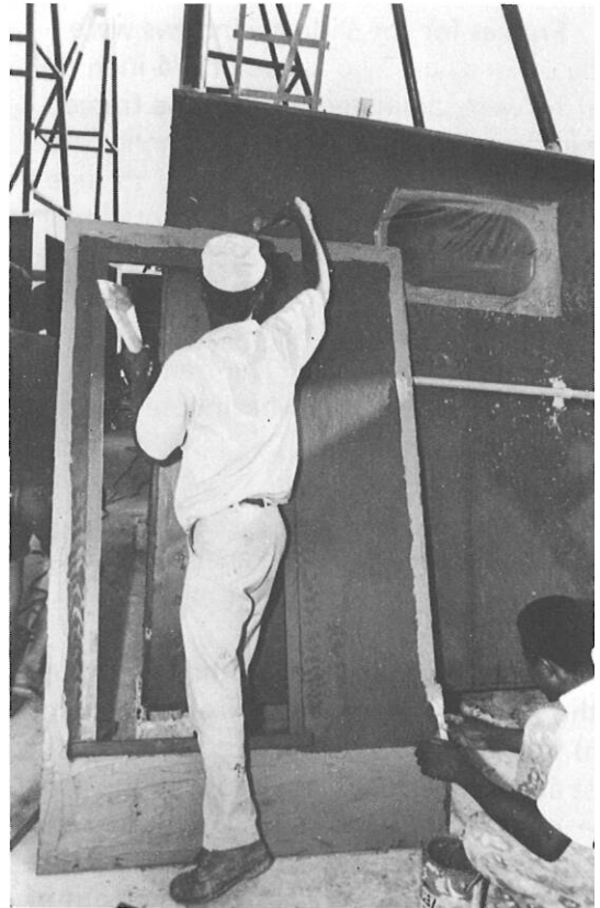
Applying bedding compound to inside face of the panel.
