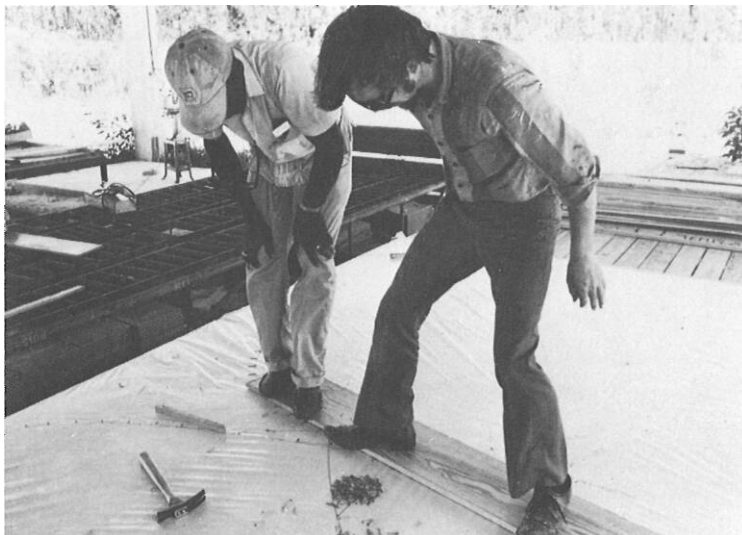
Standing on the board so that the nail heads will mark it.
