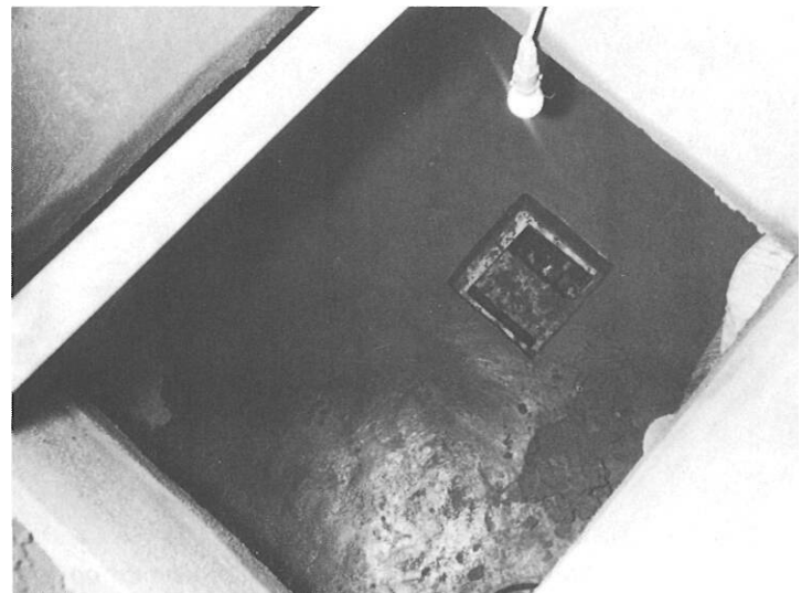
Plastering inside the fish-hold.
