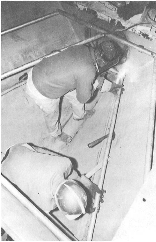
Erecting bunk supports.
