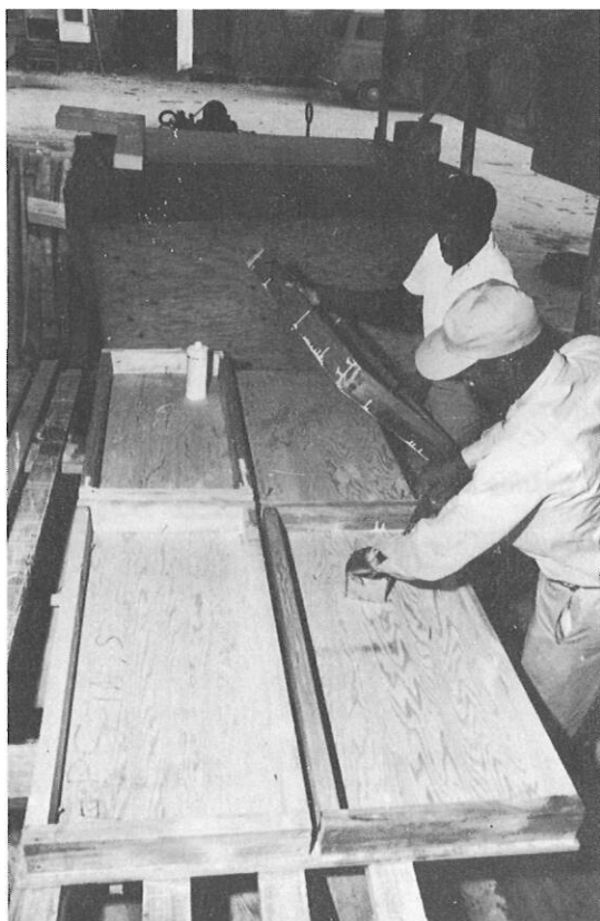
Four separate hatch frames glued to single cover.
