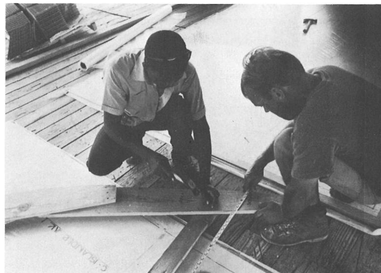
The frame measurements carefully checked before nailing together.
