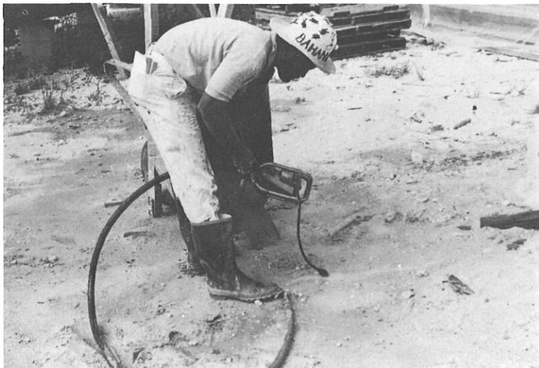
Cleaning the electric pencil-type vibrator.
