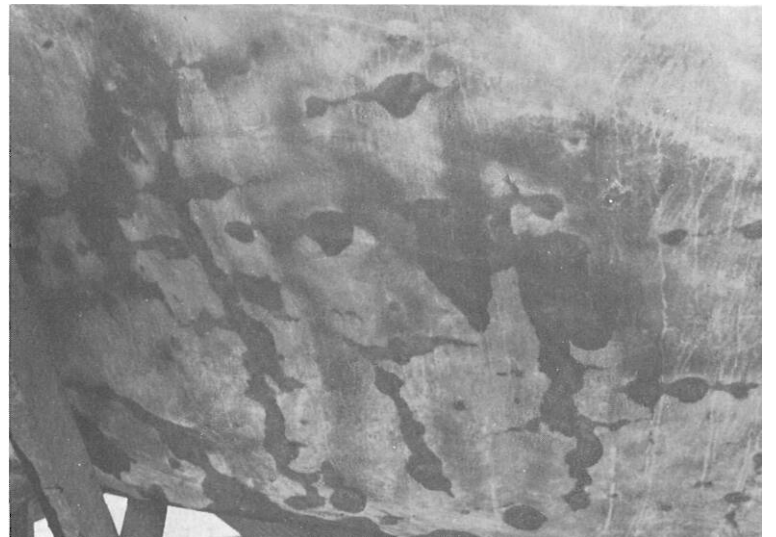
Stress cracks being sealed with the action of sodium silicate in the water.
