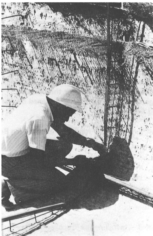
Fastening mesh to webs and stringers with hog ring staples.
