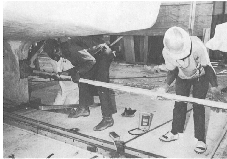
The greased propeller shaft is eased in.
