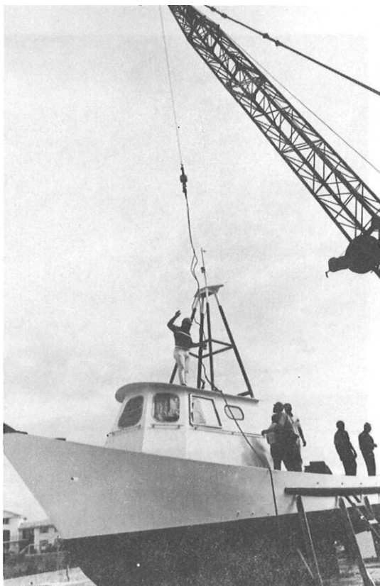
Crane released, superstructure being bolted down.
