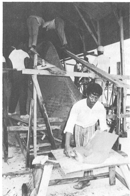
From mortar board into the hawk.
