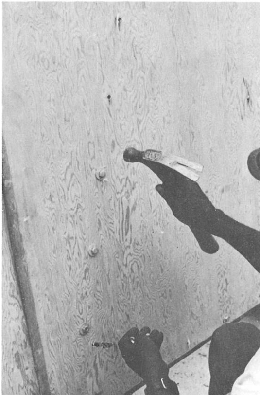
Drilled from the inside, bolts knocked through from the outside.
