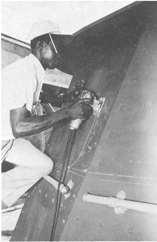
Cutting out window apertures.
