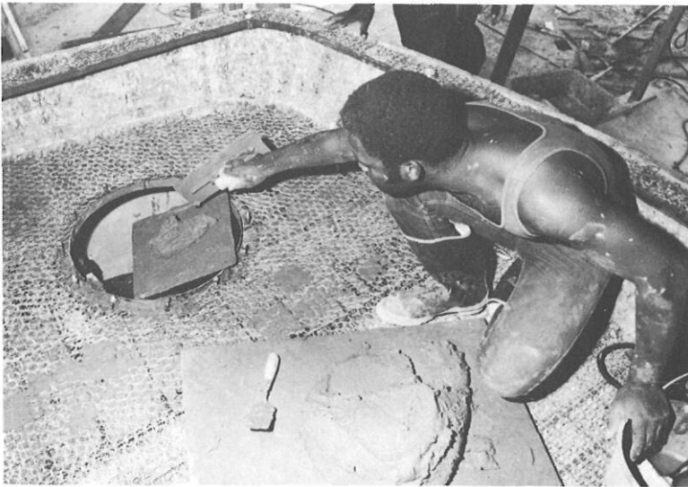
Supplying plasterer inside water tank.
