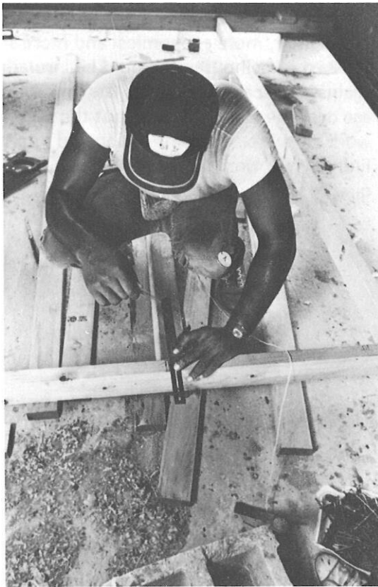
Engine room hatchway is framed first.
