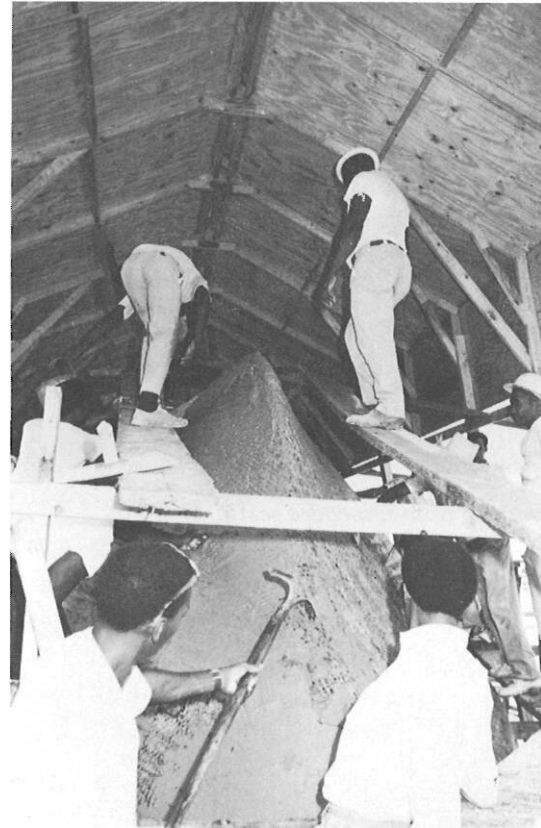
Shoveling mortar directly onto the hull.
