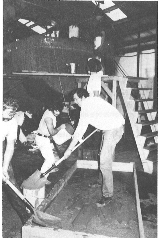
A chain of buckets being filled and passed up to the deck.
