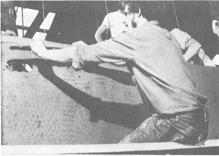
The mesh is left exposed.
