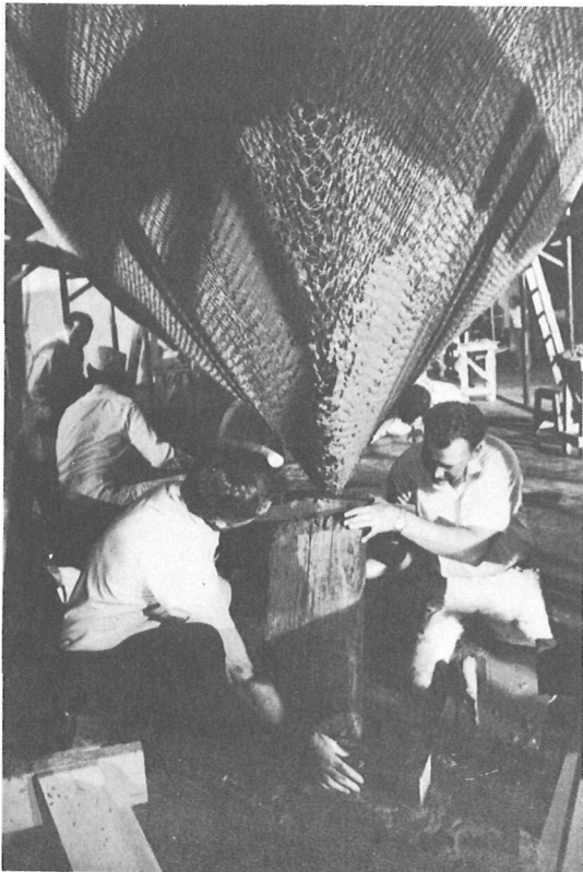
Applying mortar under keel blocks, then replacing the blocks.
