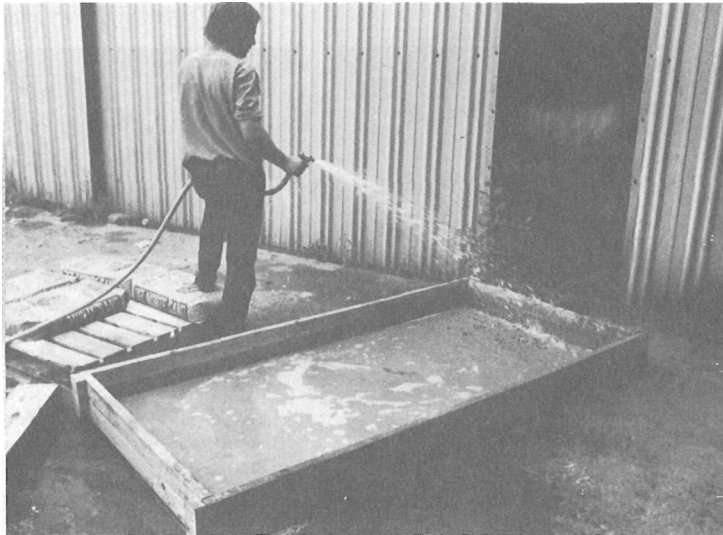
At the end of the day clean all mortar boxes, etc.
