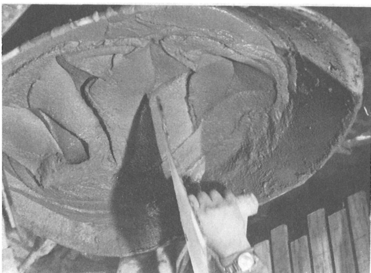
Use both the trowel and the hawk to load the hawk.
