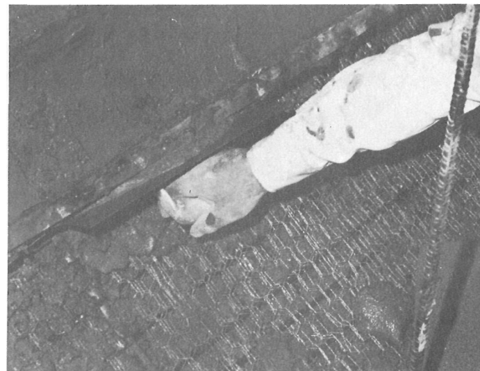
Applying mortar to a stringer.
