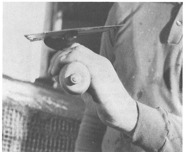
Balance the trowel in the hand.
