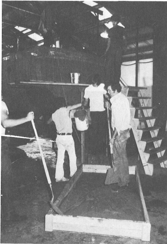
6) The mortar buckets are only partly filled. The returning buckets are dipped into a tub of water and rinsed prior to refilling with fresh mortar.
