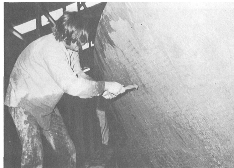
A man scraping mortar off near the bow.
