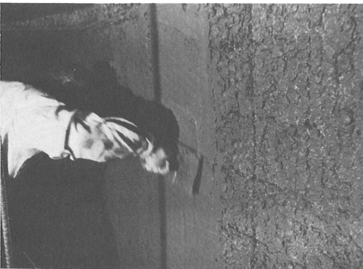
The mortar is applied at the top of the bulkheads and the plasterers work downwards.
