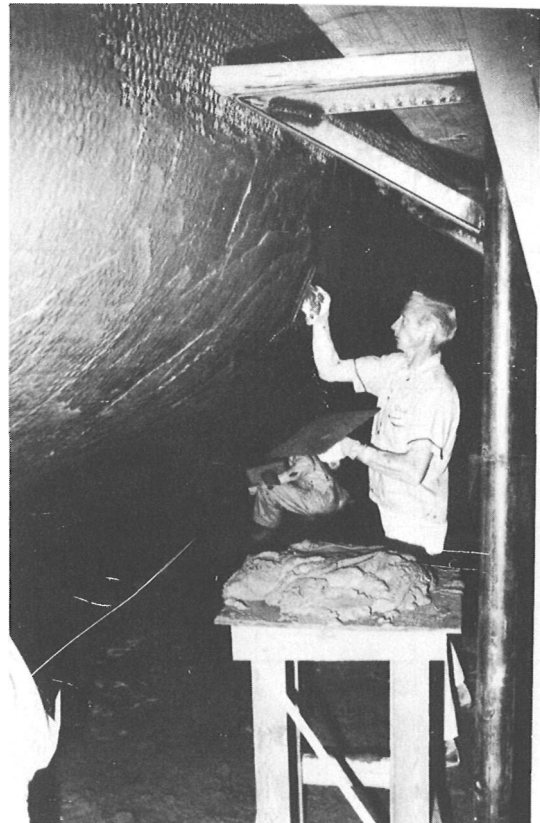
Mix consistency where no mold is to be used.
