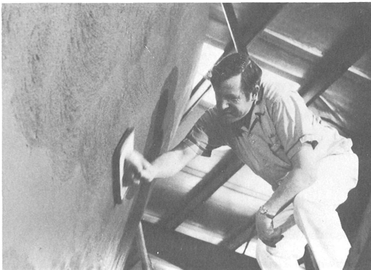
Sponge trowel being used in a circular motion.
