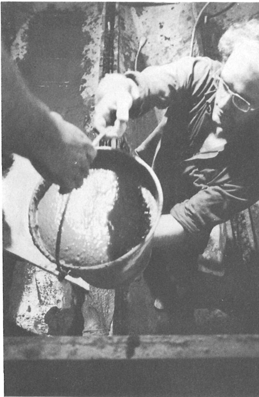
Passing mortar in for the keel.
