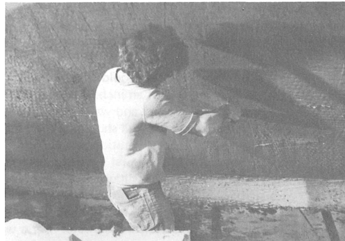
The mortar is scraped back to the surface mesh. This will enable the plasterers to control the thickness of the skin coat which is applied last.
