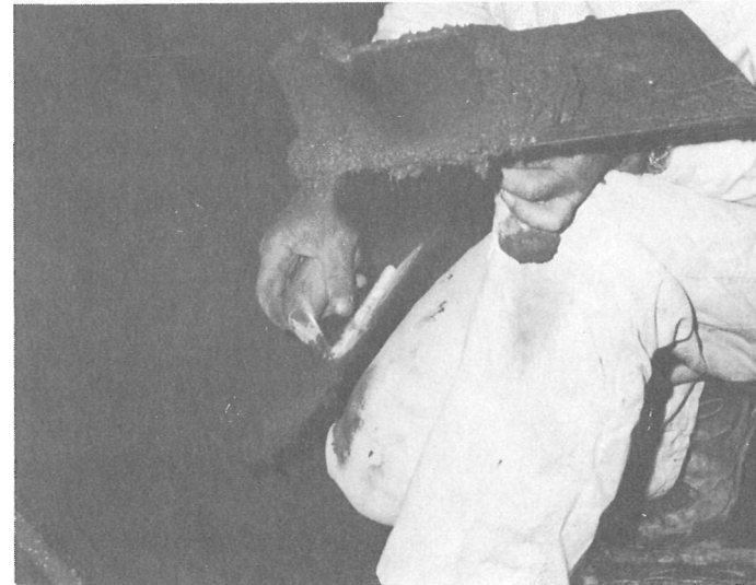
Using the hawk inside the hull.
