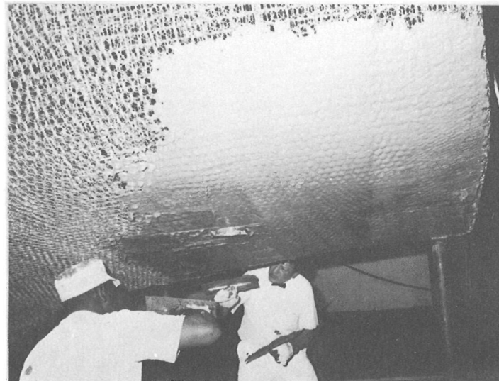
The horizontal surfaces of the hull require hard punching to get the mortar to penetrate the mesh properly.
