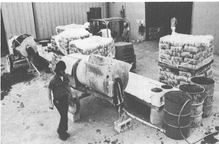
The mixers mounted on blocks prior to starting mixing. By having the mixer mounted on blocks a wheelbarrow can be filled directly from the mixer.
