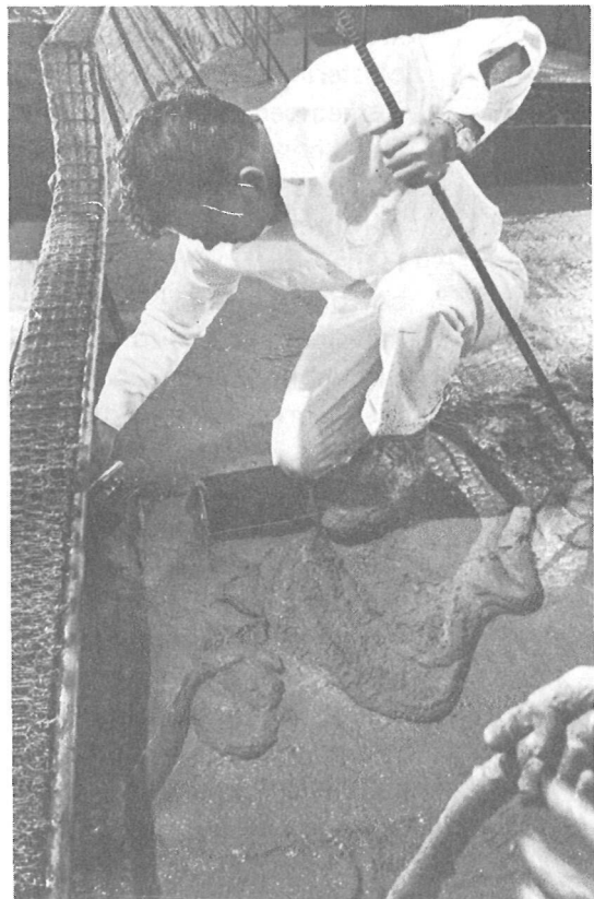
Mesh clipped in around the bulwarks cap screed.
