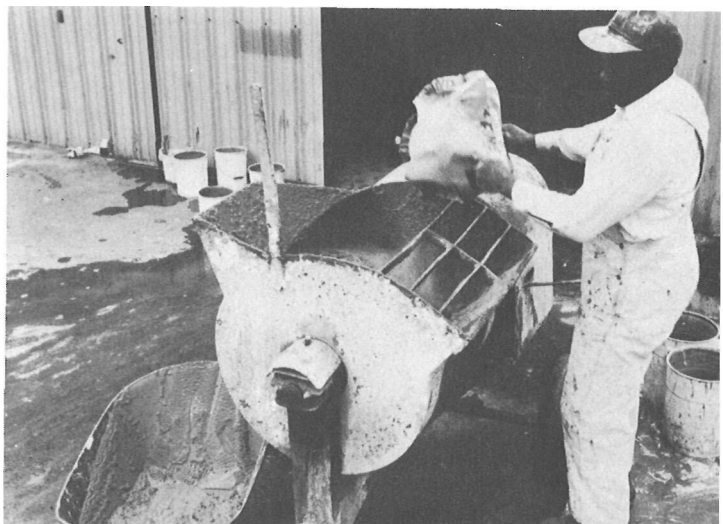
After the water and cement are in, add the sand.
