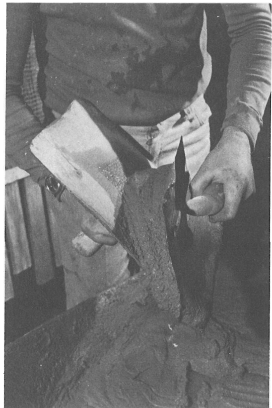
Scooping the mortar right onto the hawk.
