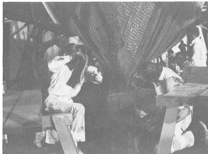
This shows the position of a plasterer's hands while effectively applying the mortar to the hull.
