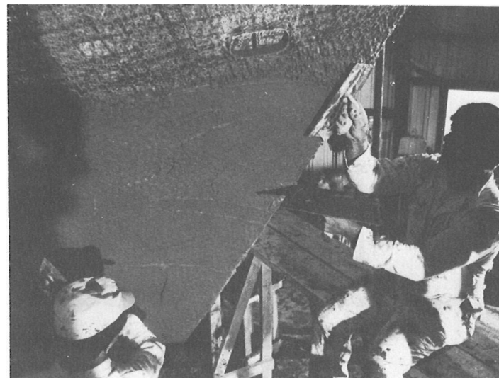
After the mortar is punched into the mesh it is spread.
