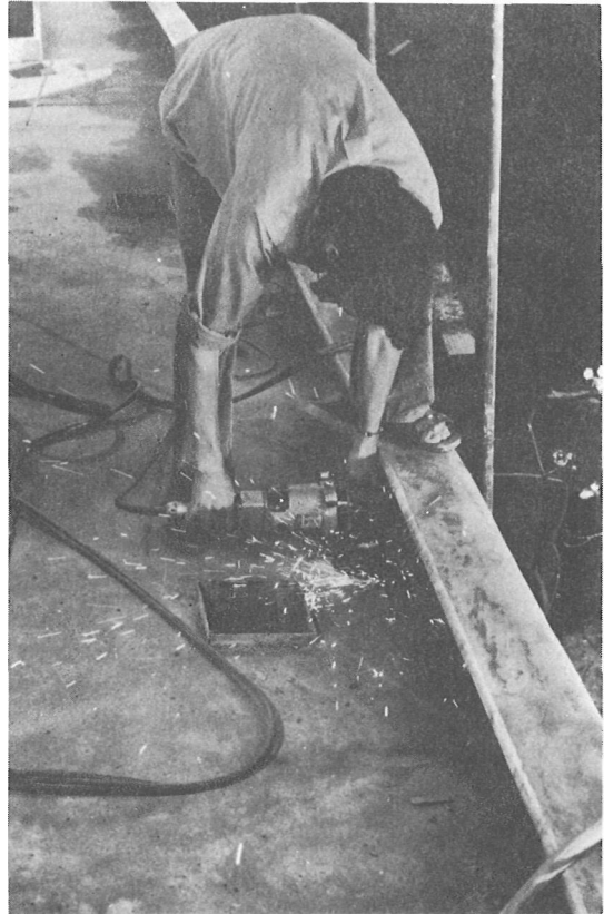
Grinding rod ends below the surface.
