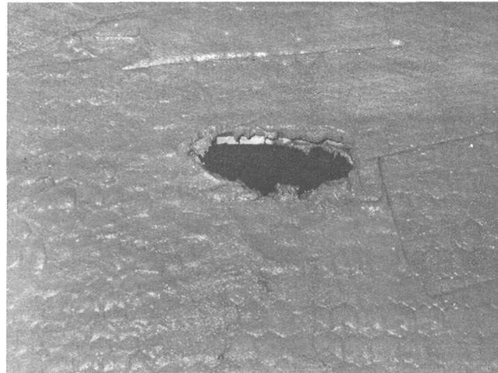
This mortar will be scraped back to the scupper screed.
