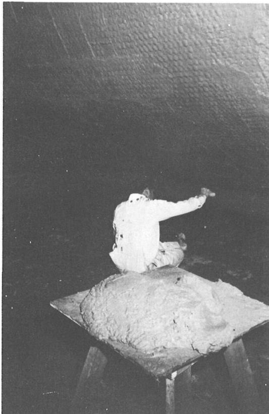
A plasterer checking over his work and applying more mortar to an area where penetration was not perfect.
