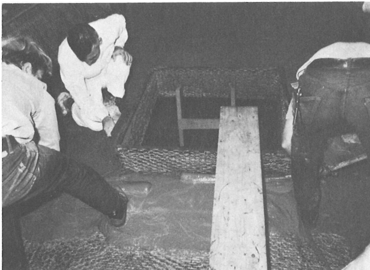
The helpers hold their feet on the vibrator heads to stop the heads from prancing around the deck and splattering mortar over the men nearby.
