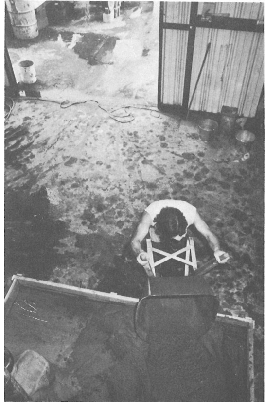
Mortar is dumped directly into holding boxes for redistribution.
