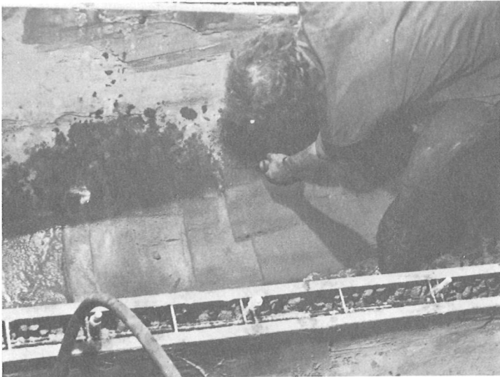
Mortar is faired into hull.
