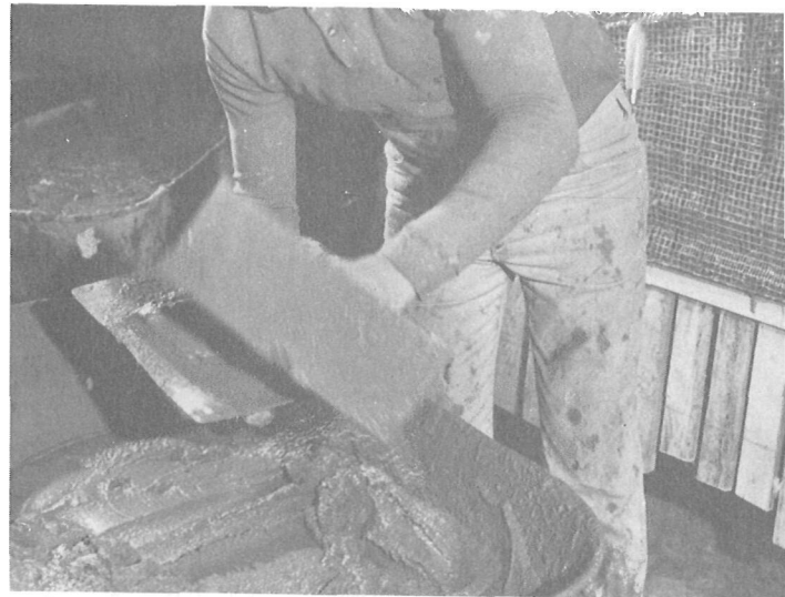
Trim the mortar off the edge of the hawk.
