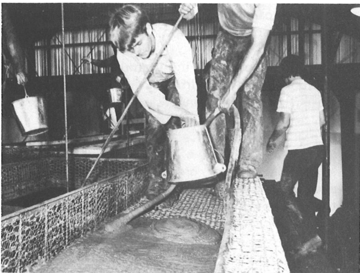
The bucket brigade dumps the mortar directly onto the deck; it is vibrated immediately.
