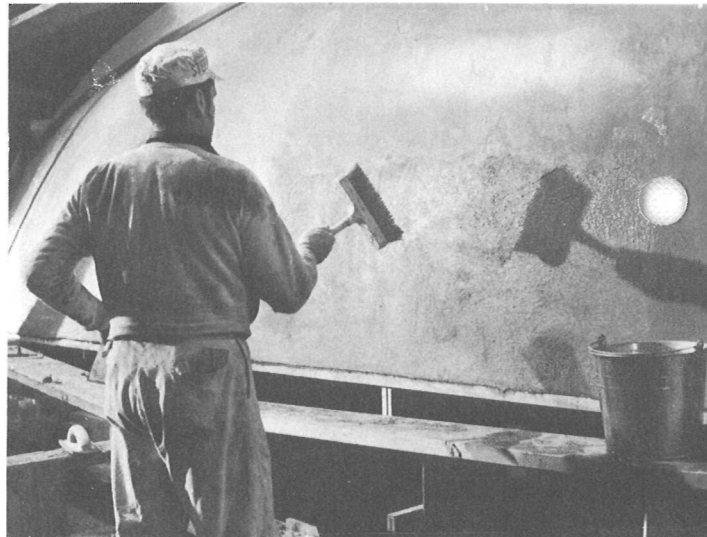
Here a plasterer is flicking grout onto the hull to assist in lubricating the surface of the mortar during final finishing. Note the edger in the plasterer's hip pocket.
