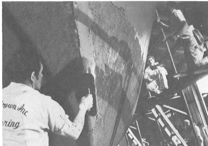
Applying the thin skin coat at the bow.
