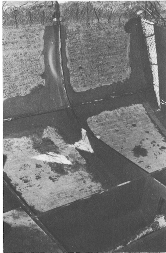
Example of cold-joint plastering, inverted wooden mold method.
