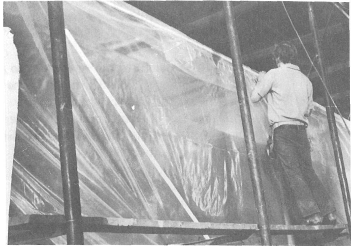
Nail battens on plastic joints.
