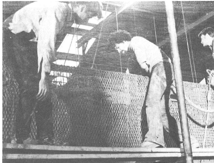
Check the edge of the deck to ensure that the mortar is penetrating this "V" joint properly.
